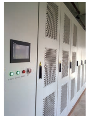
• MVD1000 for circulation water pump
