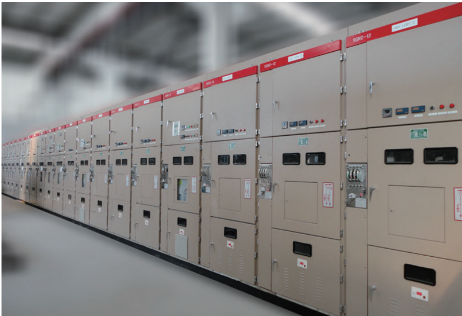
• High Voltage Distribution Cabinets
