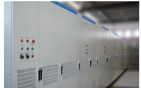
• Low voltage inverter (re-generation)
